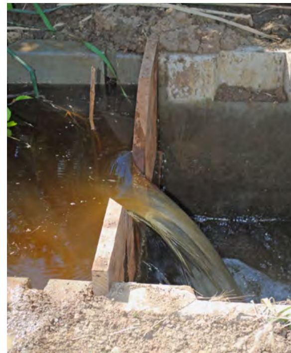
Figure 8. 90° V-notch weir.
