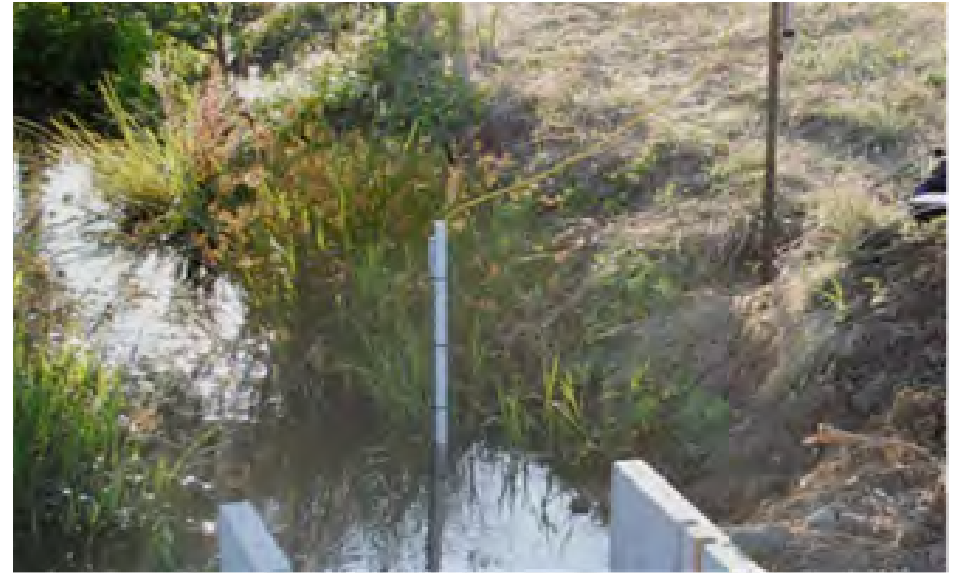
Figure 6. The pressure transducer is submerged below the water in the channel at a depth equal to the weir crest and is tied to the witness post. The transducer cable extends from the witness post back to the shoreline, where the datalogger storage device is tied to a T-post.
