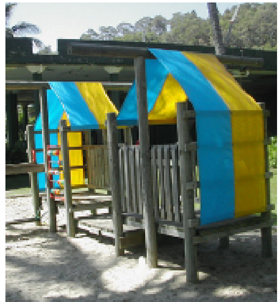
Figure 2. CCA-treated wood was used in this play structure.
