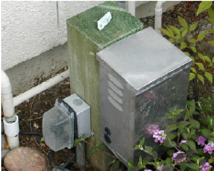
Figure 3. The typical color of CCA-treated lumber is the light green shown here. Note that the treatment identification tag is still attached to this member.
